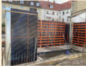
The new NeoR lightweight formwork from PASCHAL is used as formwork for the stairwell and lift core.
